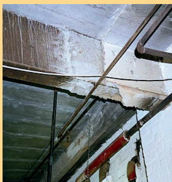
Sprayed Asbestos and Lagging.
