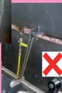
Restraining wire attached to the pipework
