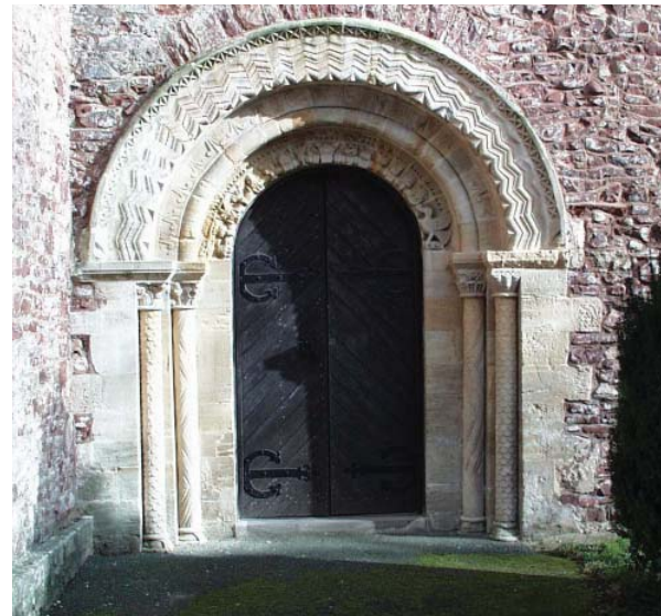
The church is built of local stone, but the decorative elements like the Norman arch are formed in Beer stone.
