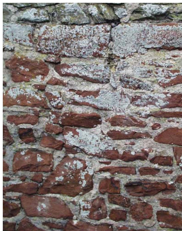
Rubble stone (tuff) wall with lime mortar and lichens.
