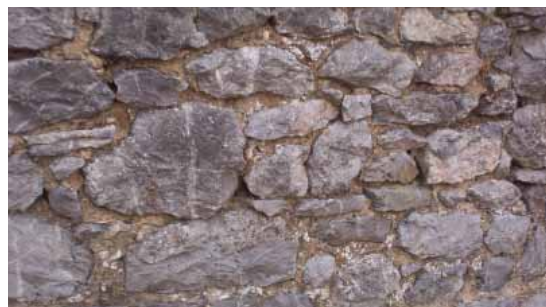
Fig 167 Traditionally pointed stone wall using lime mortar
