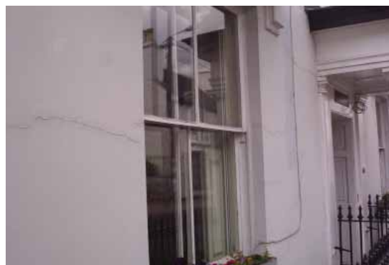
Fig 170 Shuttered timber sashes with secondary glazing fitted within reveal
