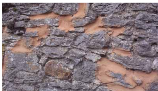
Fig 168 Poor traditional stone wall repairs using cement mortar
