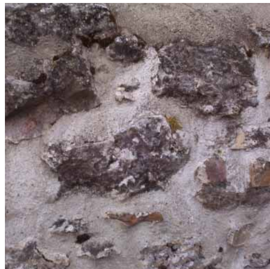
Fig 146 An example of poor stone wall construction and pointing
