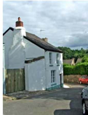
Fig 77 Chimney to gable end, 34 Clifford Street
