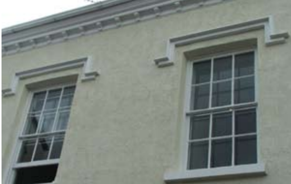
Fig 68 Window hood moulds, cornice and frieze detail to 67 Fore Street
