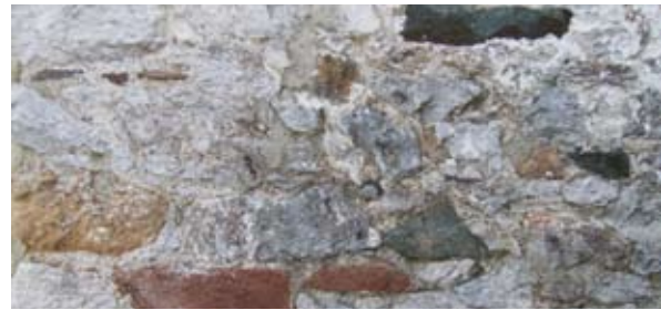
Fig 2 Irregular coursed mainly limestone wall to rear of Clifford Street, formerly limewashed
