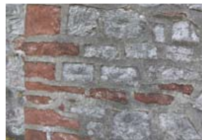
Fig 106 Cement-pointed walls to St Martin and St Mary's Church tower
