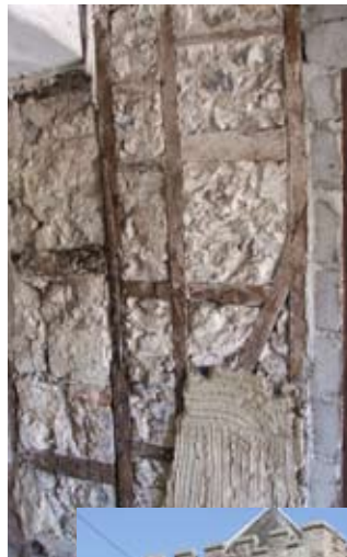
Fig 17 Timber frame exposed in cart entrance at 51 Fore Street
