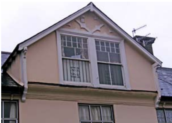
Fig 73 Jettied attic rooms with decorative timber and eaves brackets, 71-72 Fore Street
