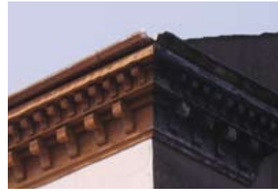
Fig 70 Eaves brackets detail to 70 Fore Street
