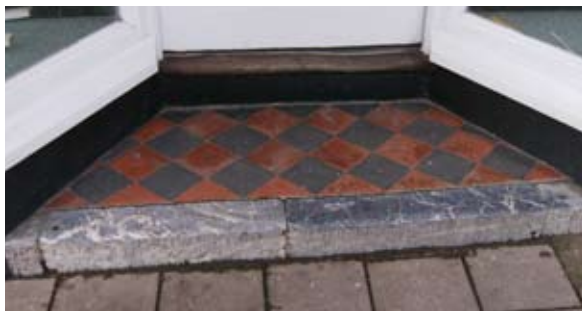
Fig 56 Geometric tile step treads, granite and limestone risers, 87-90 Fore Street
