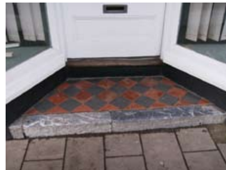
Fig 118 Geometric tile step treads, granite and limestone risers, 87-90 Fore Street
