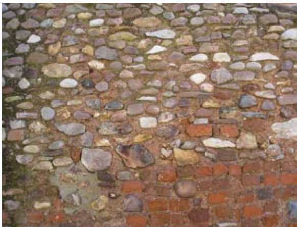
Fig 4 Uncoursed wall of red brick and cobbles
