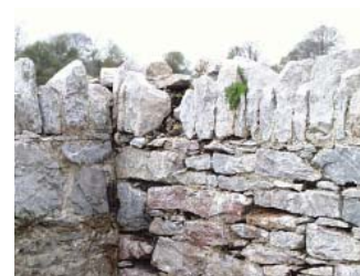
Rubble limestone walls with soldier course or 'cock and hen' capping
