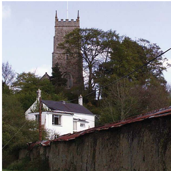
Without repair this cob wall may soon be lost
