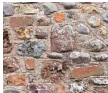
Fig 1 & 2 Rounded stones of various geological types combine with cut breccia in the walls of Holcombe.
