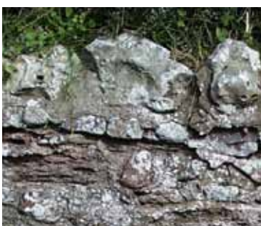
Fig 1 & 2 Rounded stones of various geological types combine with cut breccia in the walls of Holcombe.
