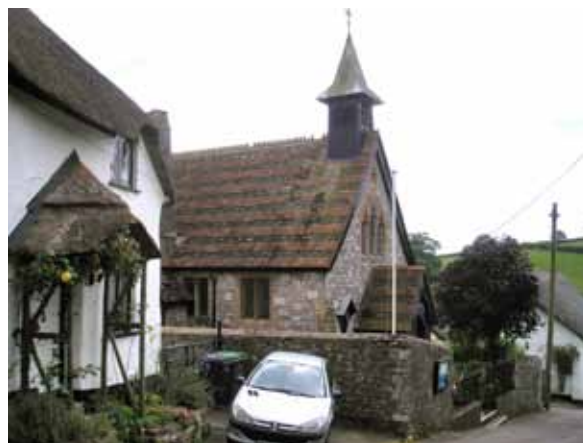
Fig 16 Thatched cottages of stone and cob construction, built close to the road, are typical of historic Holcombe.
