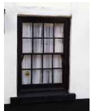
Fig 27 Typical sliding sash windows
