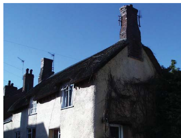
Rendered and limewashed walls with thatched roof epitomise the original building forms in Ide
