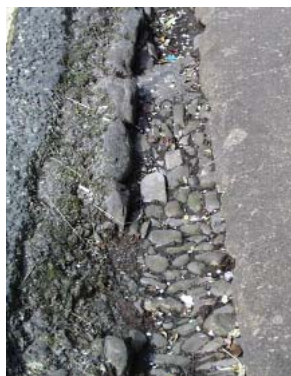
Cobbling should be repaired and, where possible, reinstated
