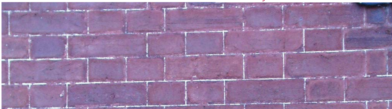
Tuck-pointed brickwork
