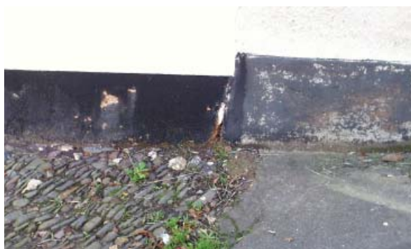
Too often traditional surfacing has been obliterated by tarmac or concrete. Note how the cobbles efficiently channel water away from the base of this wall, as well as adding visual interest to the floorscape.
