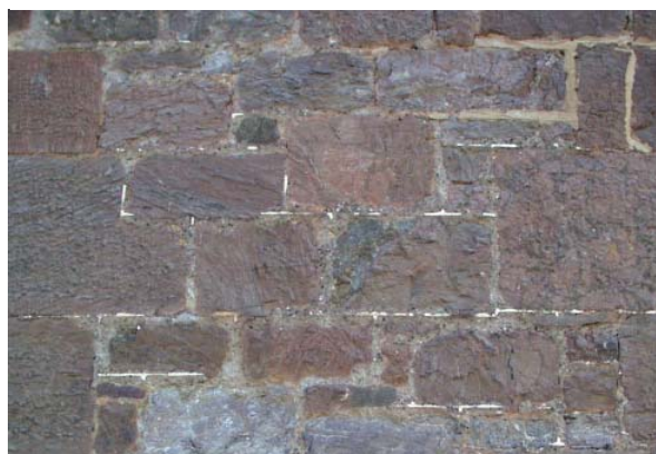
Tuck-pointed Trachybasalt
