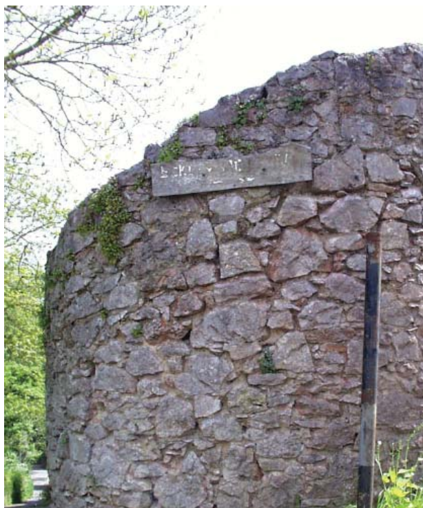
Rubble limestone walls often form enclosure
