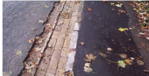
Fig 38 Buff brick gutter lining
