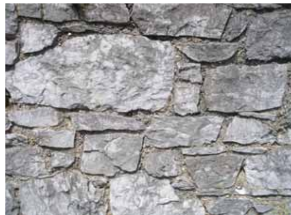
Fig 3 Grey limestone used on boundary walls, random rubble bond
