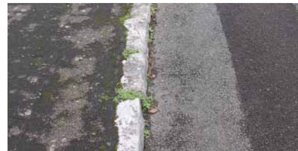
Fig 40 Limestone Kerb
