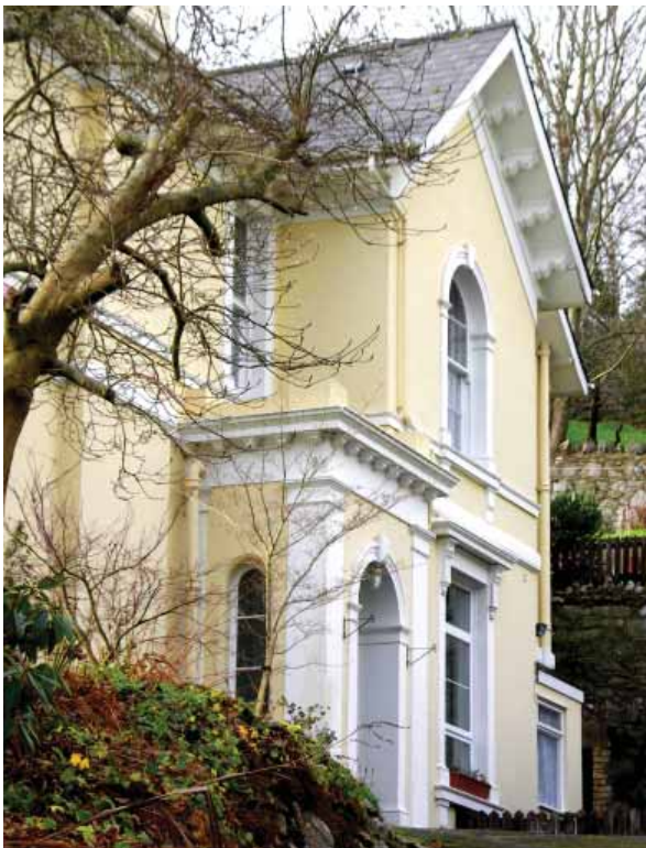
Fig 58 Typical rendered walls with slate roof
