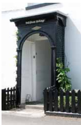
Fig 29 Hill View, hood with sides added
