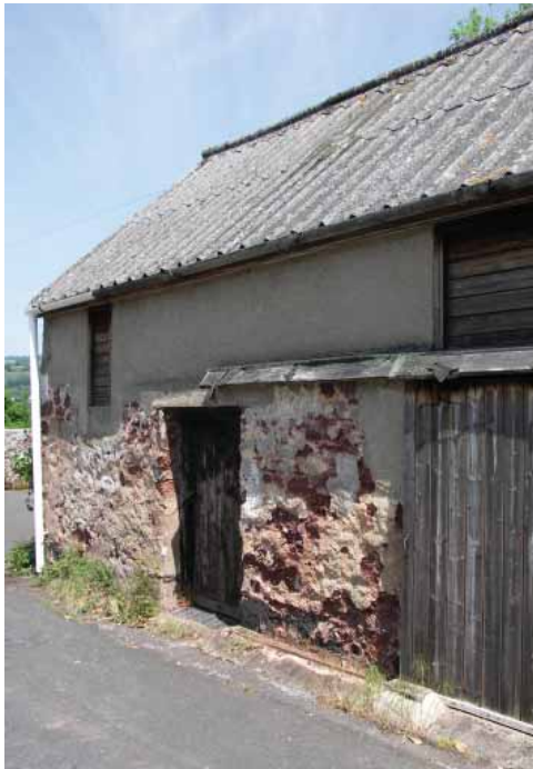
Fig 37 Exposed stonework in a farm building
