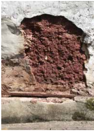
Fig 32 Exposed cob of outbuilding
