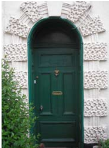
Fig 64 Vermiculation around door, Bridge Road
