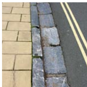
Fig 27 Limestone kerb and gutter
