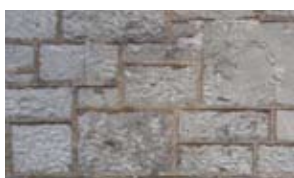
Fig 1 Historic coursed limestone used on higher status buildings.
