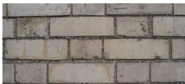
Fig 3: Buff bricks in Flemish Bond
