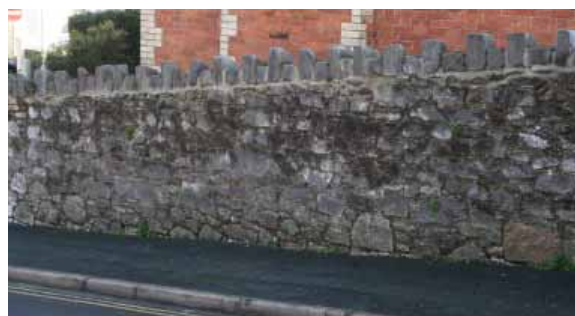
Fig 55: Typical limestone boundary wall with cock and hen capping.
