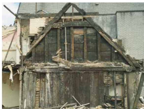
Fig 9: Remains of 16th century roof and incorporated in a later building, 25 Wolborough Street
