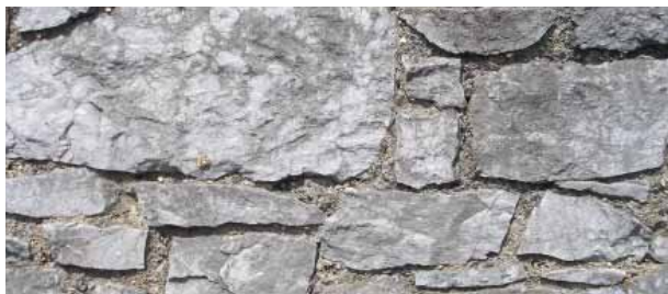
Fig 1: Limestone Rubble Bond
