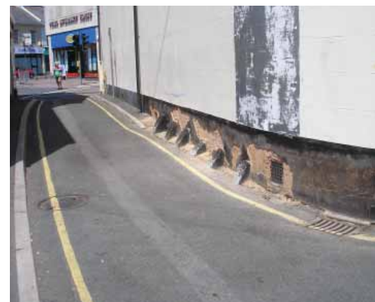
Fig 67: Rubbing stone at Hopkins Lane to prevent cart damage to buildings
