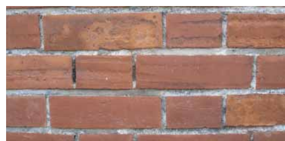
Fig 4: Red bricks in Flemish Bond
