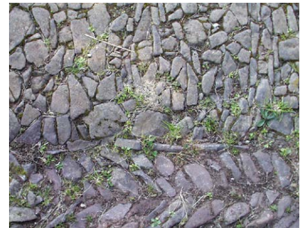
The local basalt is a very durable material which is good for cobbling.
