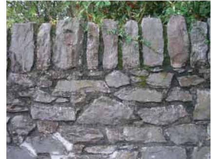
Grey limestone used on boundary walls, random rubble bond.
