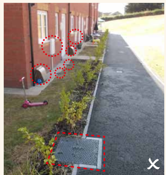
Poorly co-ordinated and integrated services undermine design quality from the outset and are costly to rectify
