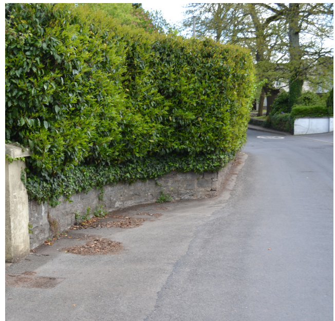
Low stone retaining walls are frequently found topped with hedgerows to overcome level changes where plots meet public areas
