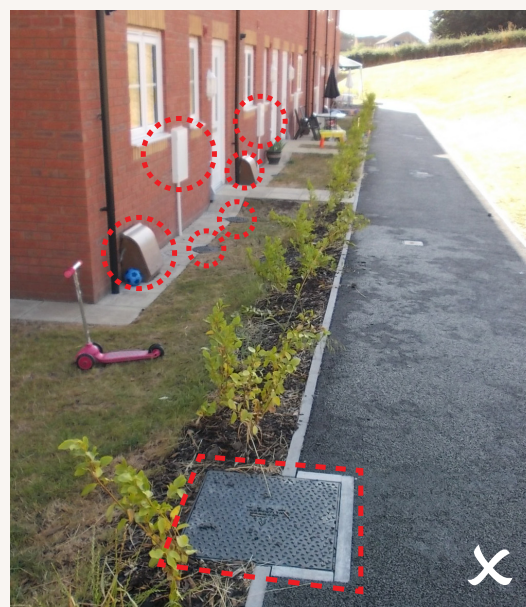
Poorly co-ordinated and integrated services undermine design quality from the outset and are costly to rectify
